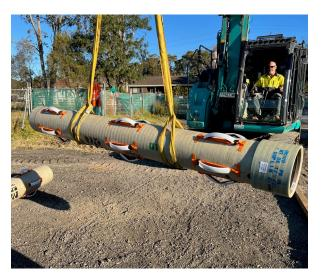
At each end of the installation, centralizers should be placed a distance of half of the linear spacing from the end of the pipe to support the overhanging section of the pipe. In most cases this will be **0.5m.**
